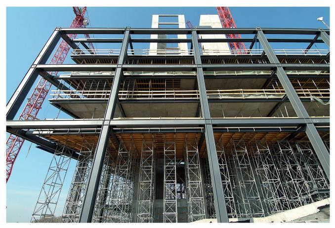
High load capacity of 200 kN per tower even with small base dimensions (1.00 m x 1.00 m)
