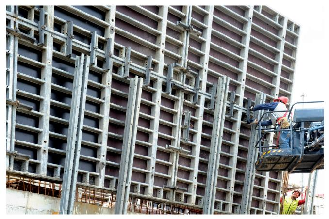
A special solution: Facade walers are used to ensured back anchoring of the horizontal loads and to enable the exact alignment of the MANTO formwork in a desired inclined position.
