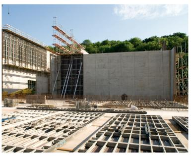
By using facade soldiers, the 16.73 m high walls of a terminal were shuttered in two pouring cycles instead of three.
