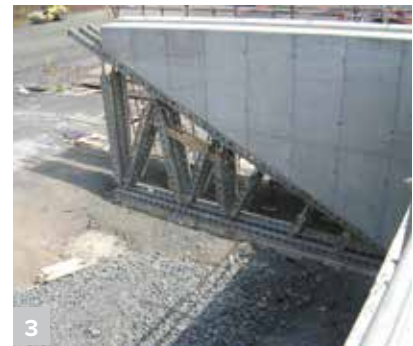
3 Load capacity of up to 100 kN – concrete pressures up to 80 kN/m 2
